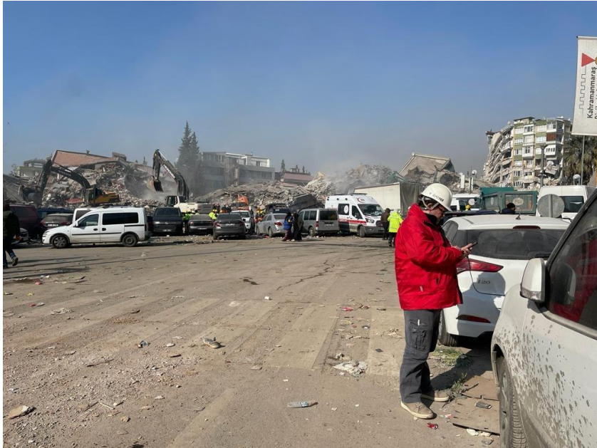
MI assessing the damage in Kahramanmaraş
